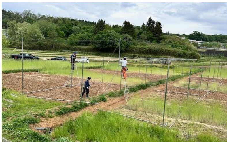
Figure 14 [Test Plant Installation Scene ② Assembling the Prepared Mounting Frame: April 2024]
