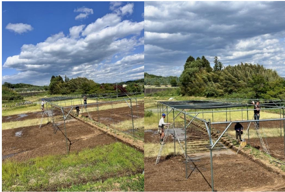
Figure 15 [Test Plant Installation (3): Attaching Dummy Panels – April 2024]
